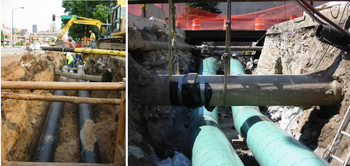
Figure 4-9: Installation of Distribution Pipe around Existing Utilities
