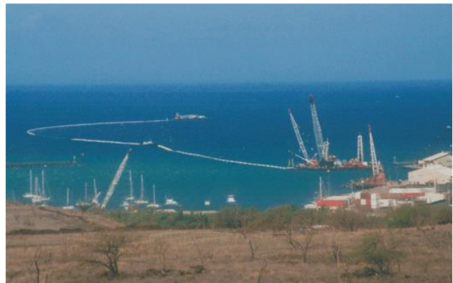
Figure 4-3: Controlled submergence of an HDPE pipe designed by Makai.
