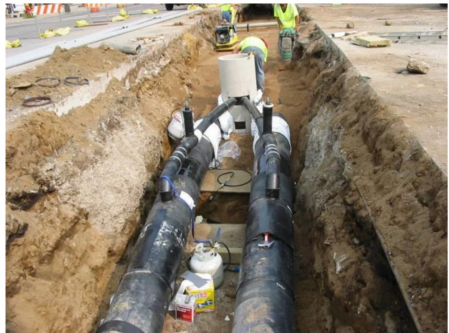
Figure 4-7: Distribution Pipe Installed under a Roadway
