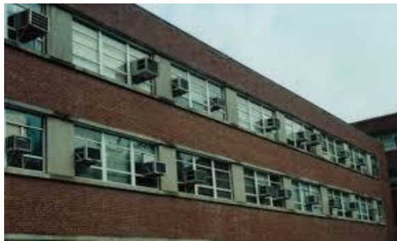
Figure 6-9: Example of Window Unit Air Conditioners
