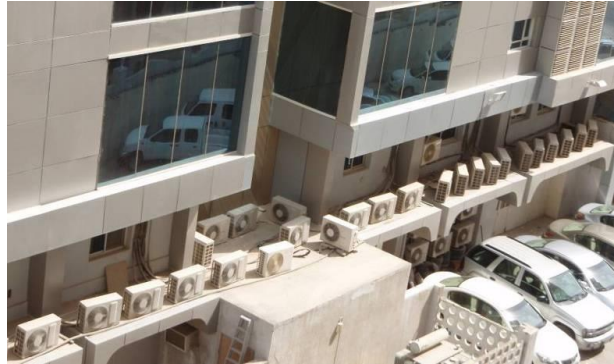
Figure 6-8: Example of Mini-Split Air Conditioning Systems
